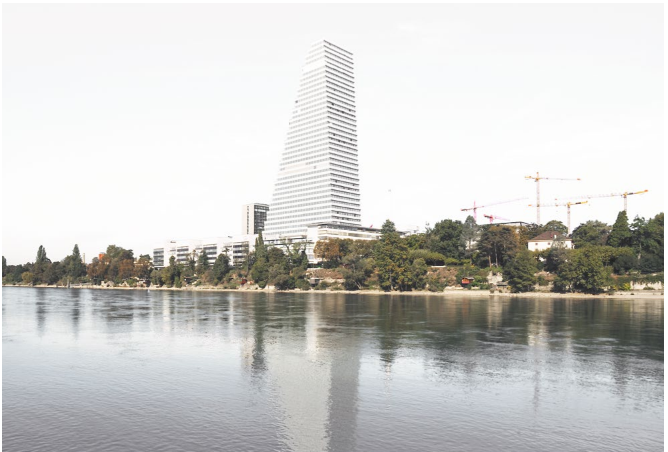
Roche-Turm (Bau 1) Basel
